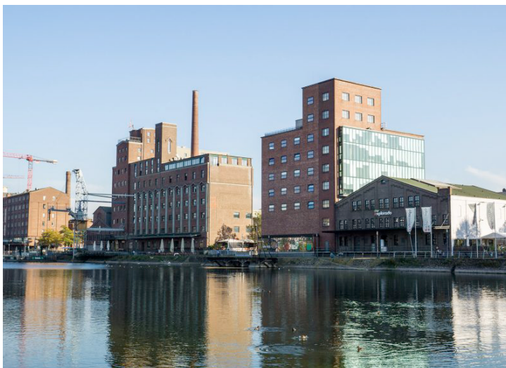
Start Port Head office
